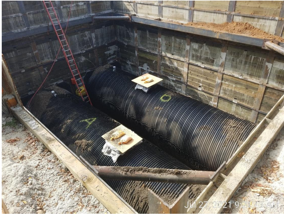
Retention Tank Installation
