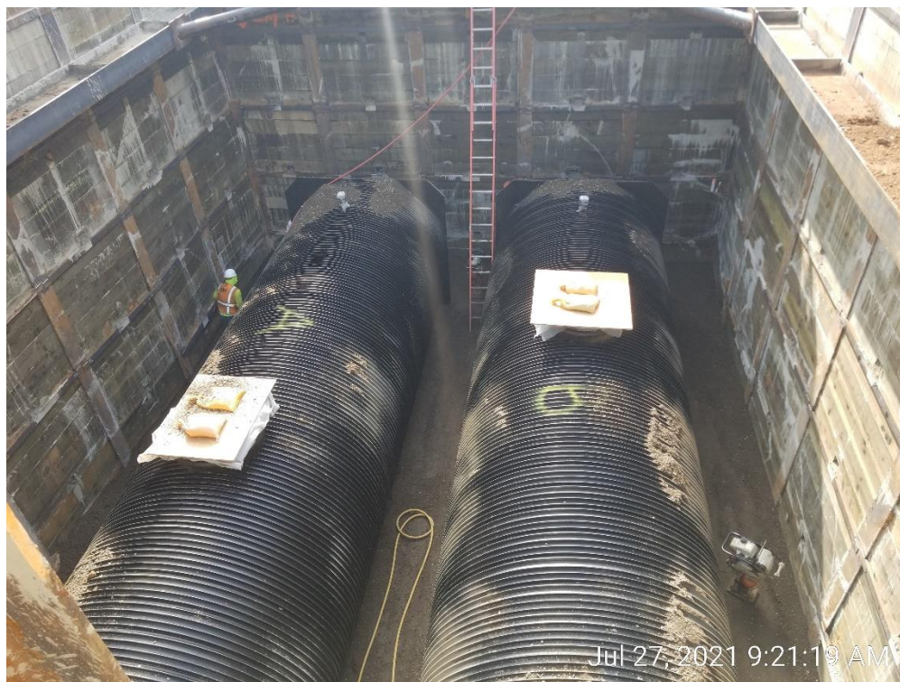
Retention Tank Installation
